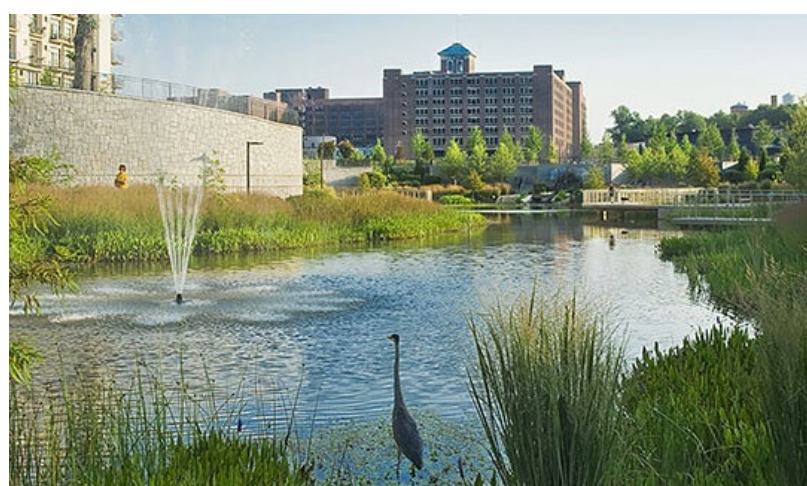
CLEAR CREEK STORMWATER BASIN | ATLANTA, GA | STEVE CARRELL
